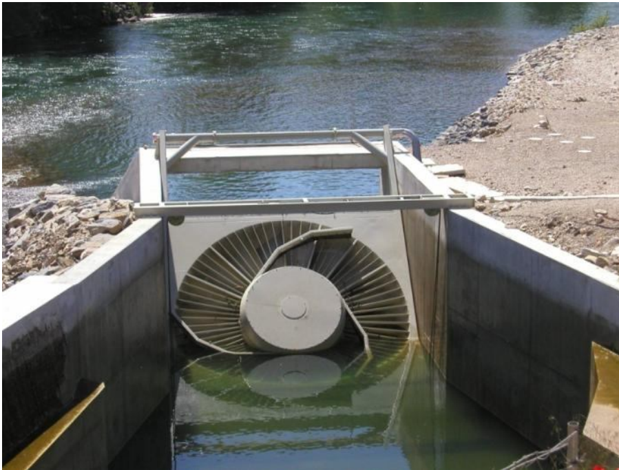
Upstream view of the VLH in the empty inlet channel
