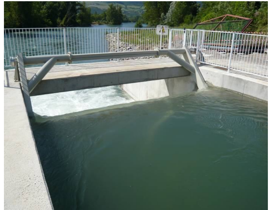
VLH in Operation
